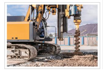
The structures required the construction of a considerable amount of Continuous Flight Auger foundations<sup>2</sup>. Balfour Beatty engaged Van Elle to carry out the piling works. The agreed total price for these works was £1.239m.
